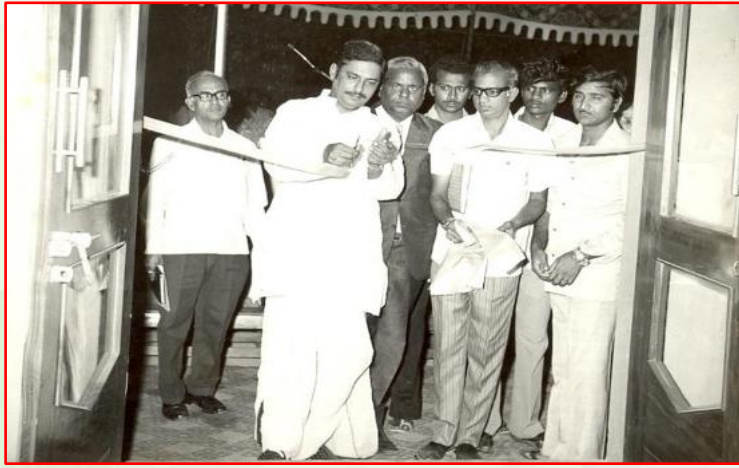
Inauguration of BHEL ECCS in the year 1976.
